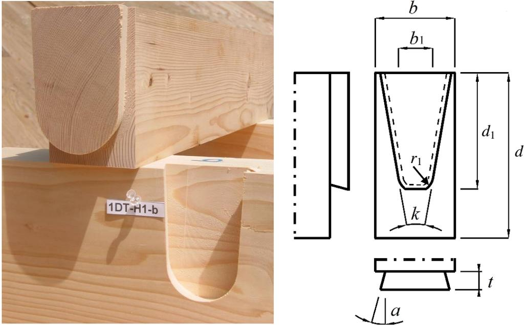
Figure 1 – Rounded Dovetail Joint: photo (left) and geometric parameters (right)
