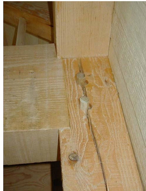
Figure 1 Splitting failure
